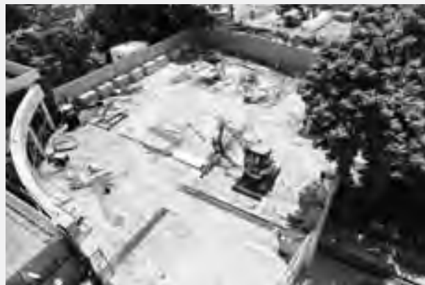
An aerial view of the new building's construction site
